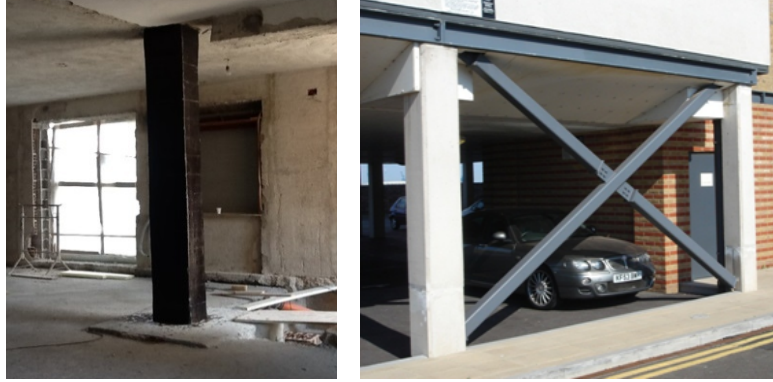
Fig. 2: Example of local confinement (left); and concentric steel bracing (right)
