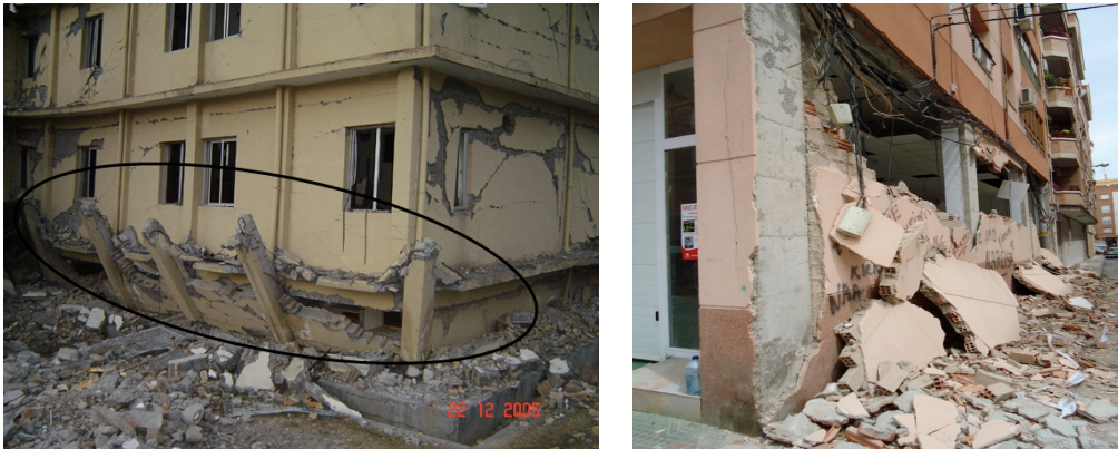
12 Fig. 1: Example of brittle mechanism (left); and ductile mechanism (right)
